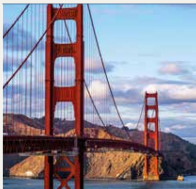
Golden Gate Bridge
