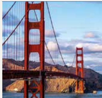
Golden Gate Bridge
